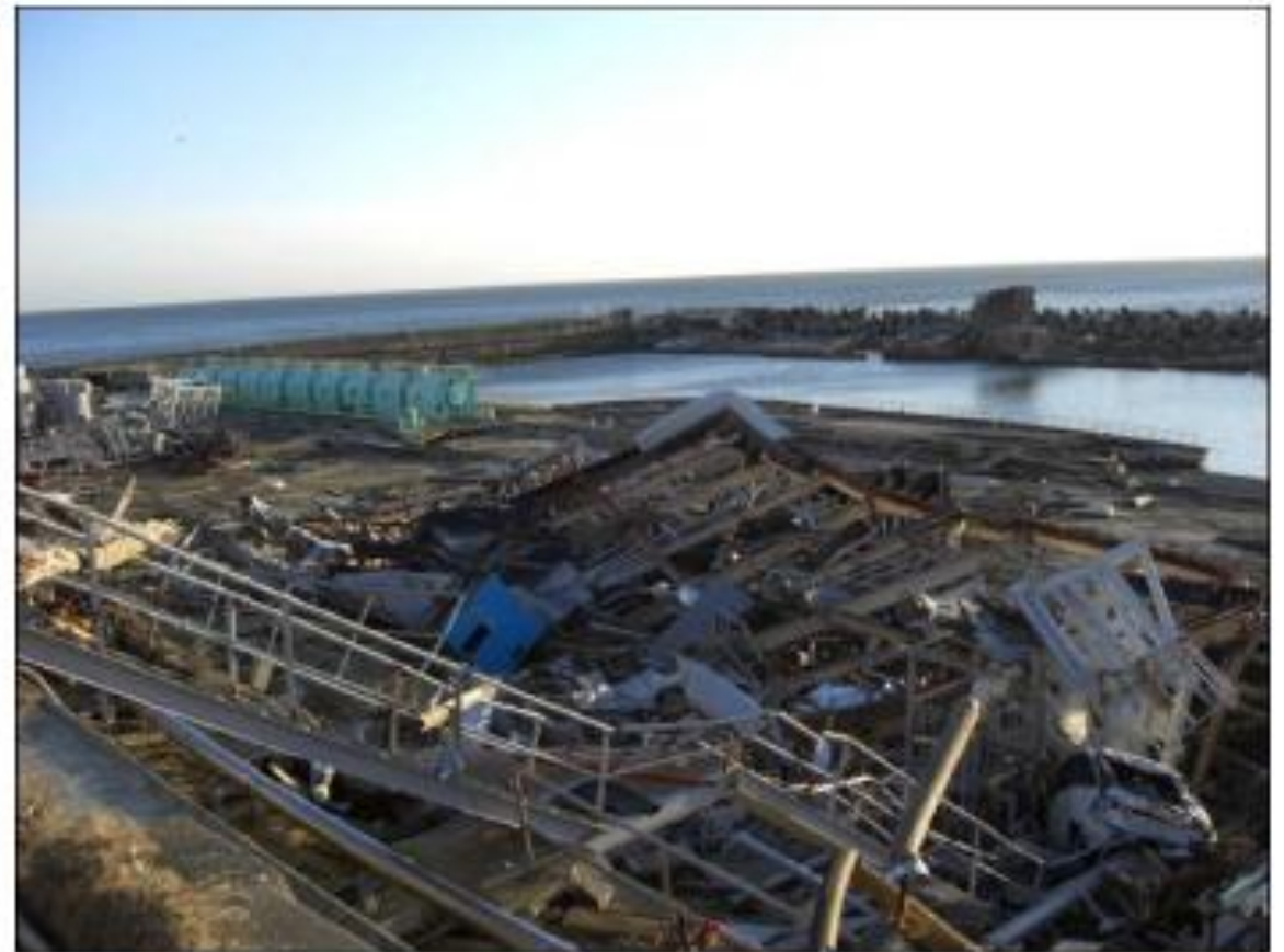
Unit 5,6 Intake Screen Area
