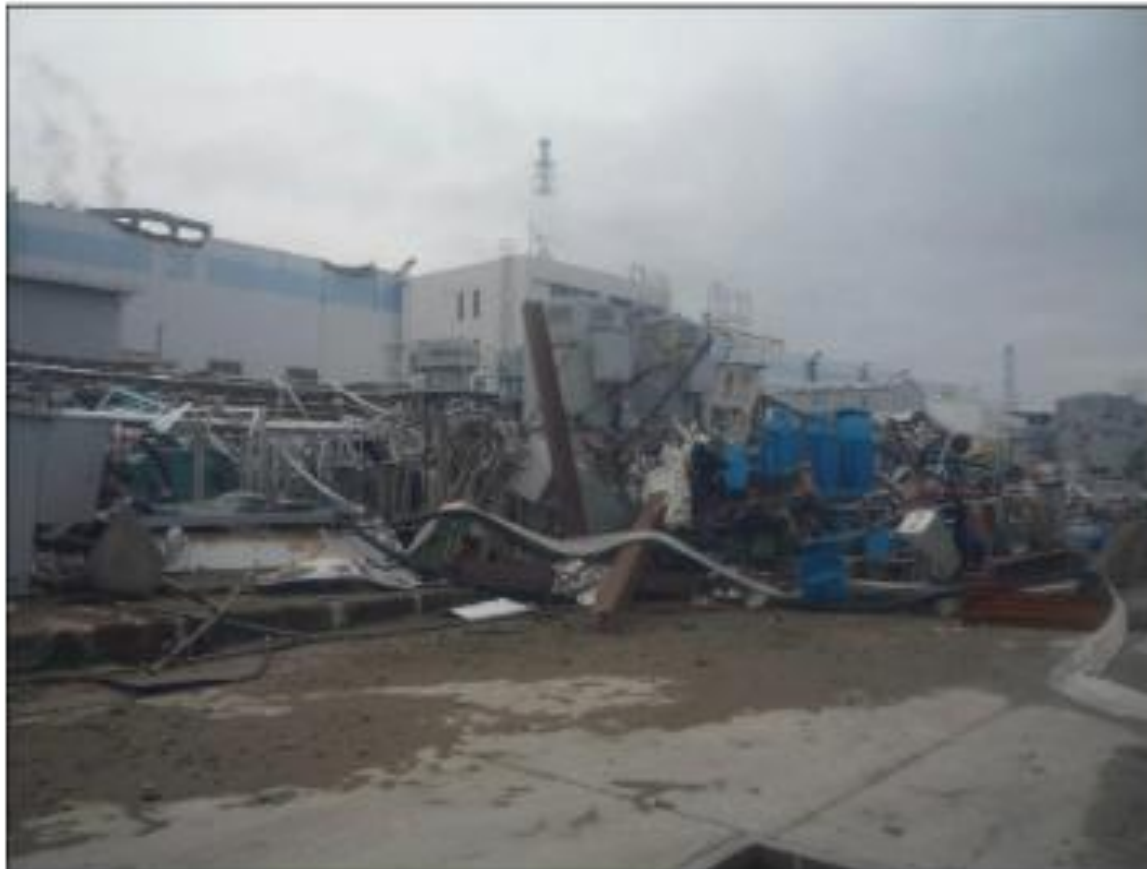
Unit 3 Sea Pump Area
