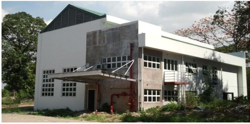
L5 Laboratory Building (Fire Laboratory)
