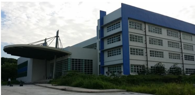
Office and Classroom Wing (OCW) Building
