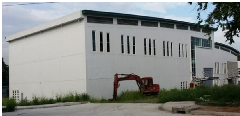
L1/L2 Laboratory Building (Structural Engineering and Construction Engineering Laboratories)
