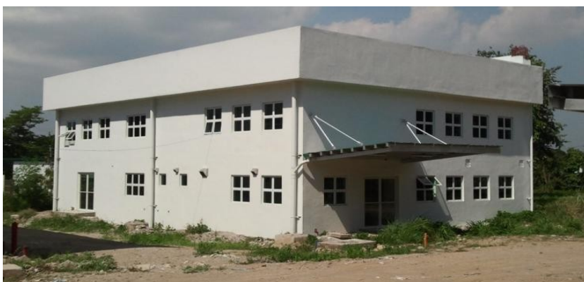
L3 Laboratory Building (Geotechnical Engineering Laboratory)
